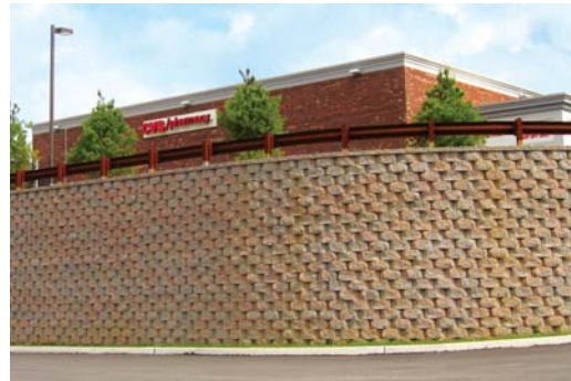
A Mesa Retaining Wall supports the CVS Pharmacy at the Brookworth Plaza project.
