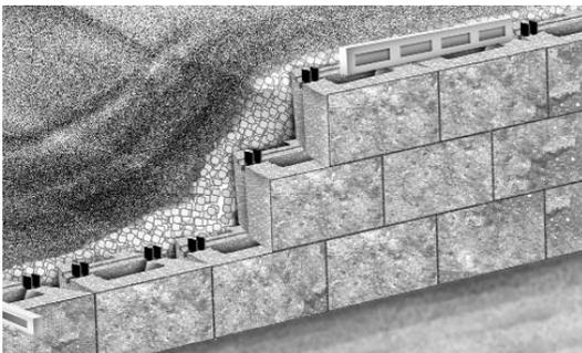
As subsequent courses of Mesa Units are placed, it is important that the units remain level from front to back and side to side. This level should be checked as each course is placed. If the units are more than 1/8-inch out of level from front to back or side to side, or if the units are not level from back to front, they should be brought to level by grinding and/or shimming (see Figure 1 to the right and Figure 2 on page 8).
