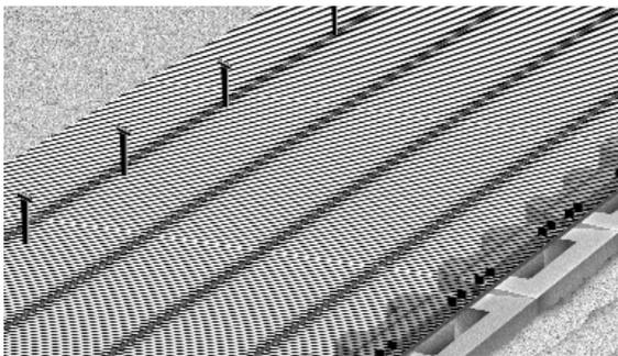
can be gradually sloped. Remove slack from the geogrid by pulling it taut, and then anchor it using stakes and/or rods. The stakes used to position the tail of the geogrid can be withdrawn once the fill has been placed and then reused on subsequent lifts. Optionally, a pitchfork can be inserted at the tail of the geogrid and slack removed by prying until the fill has been placed on the geogrid. The removal of the slack from the geogrid prior to fill placement
