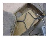
7. Wires will be rejoined and lights attached using the connectors. Examine the connectors and note that there are three holes in each. Take the ribbed side of one end of the
