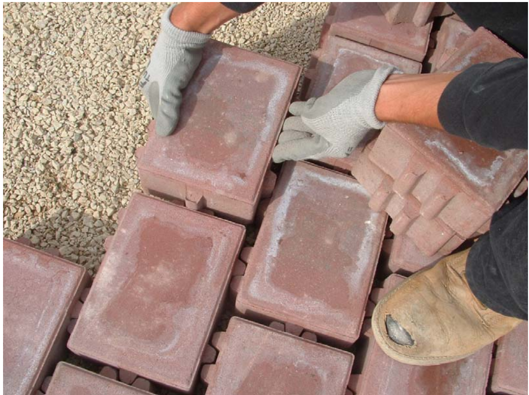
Eco Paver installation over pea gravel utilizing interlocking fingers
