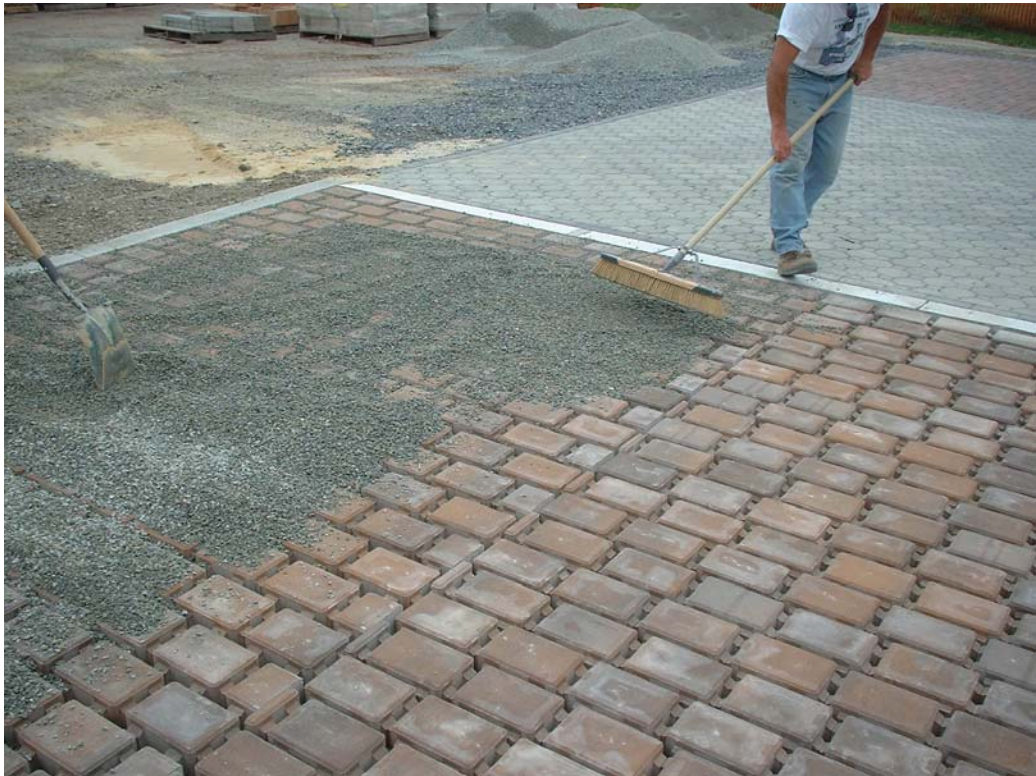
Pea gravel placement between Eco Paver units
