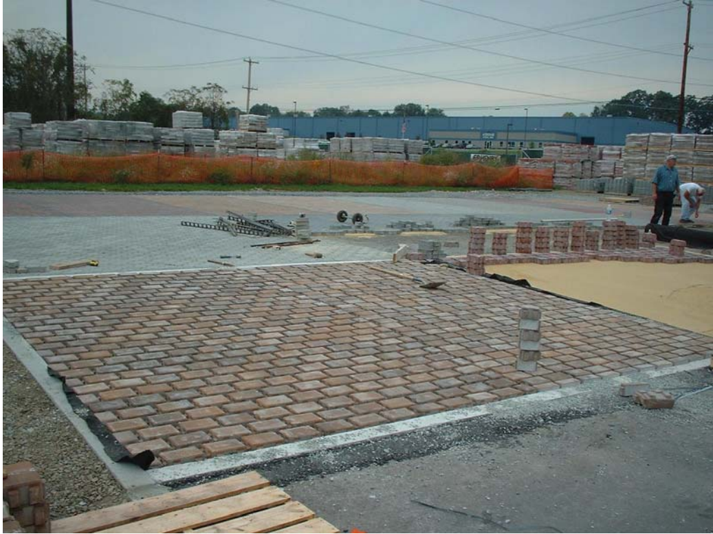
2A stone subbase Eco Paver pad
