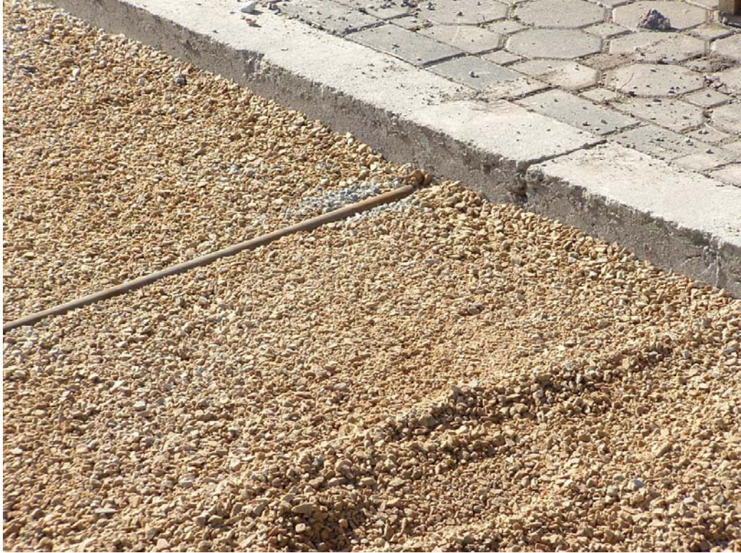
Eco Paver pea gravel leveling pad
