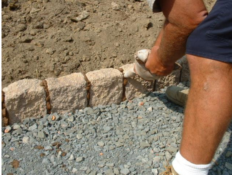
Mortaring joints with Mortar Bag
