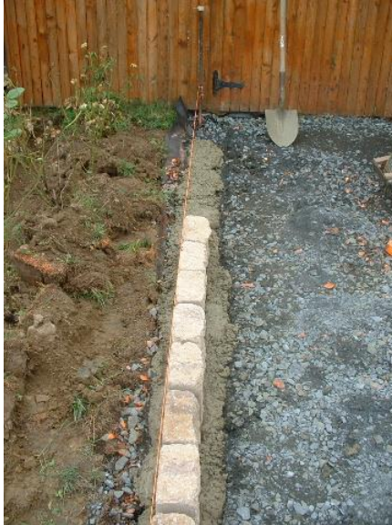
String line for aligning the block
