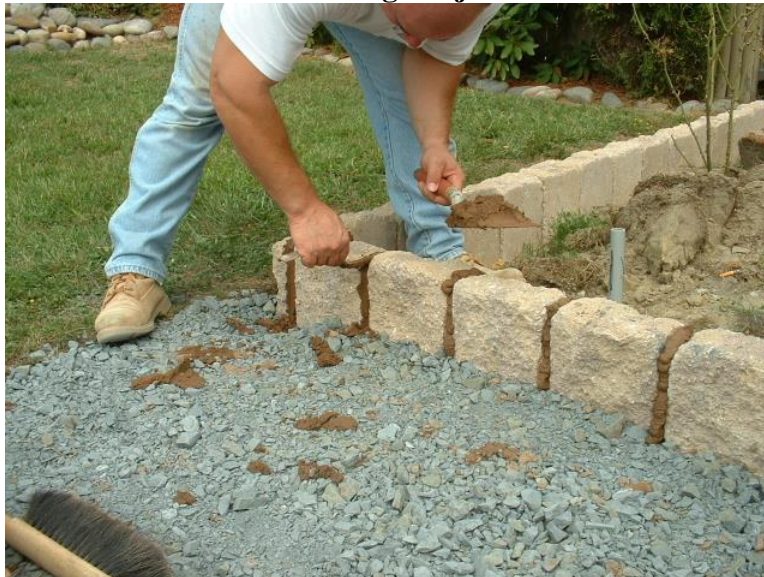
Tooling the joints
