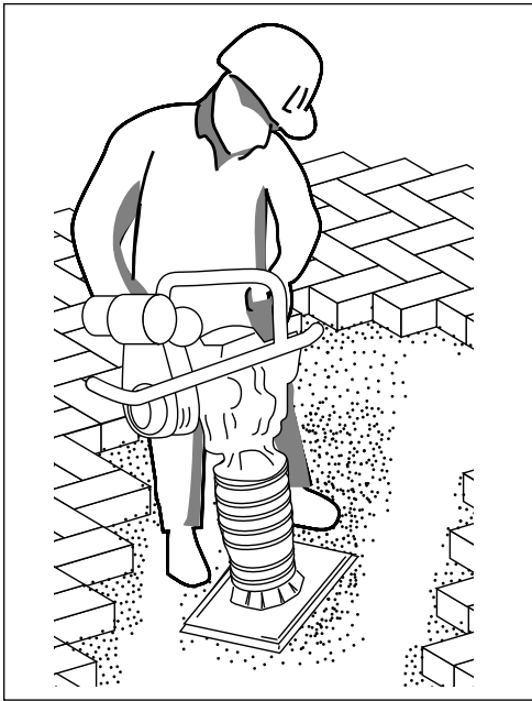
Figure 10. Compaction of the base in 2 to 4 in. (50 to 100 mm) lifts and monitoring density with a dynamic cone penetrometer or a nuclear density gauge are essential to minimizing settlement.
