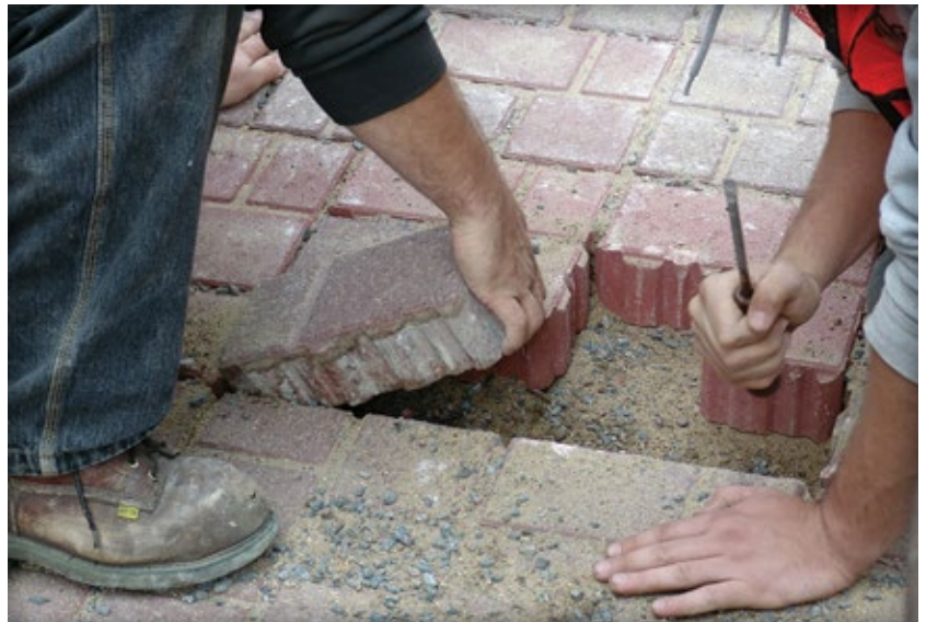
Figure 7. Pulling out a paver by the short end provides greater leverage and makes extraction easier.
