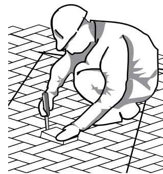
Figure 4. Prying with a screwdriver and pulling the paver out.
