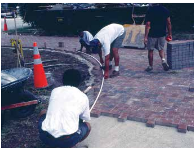
Figure 14. Marking pavers for saw cutting. The cut pavers are carefully removed and edging is placed against the pavers.
