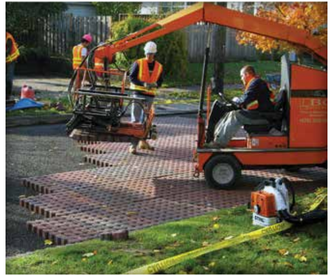
Figure 27 and 28. Mechanical equipment accelerated installation of a parking lot in Illinois and a street in Oregon.
