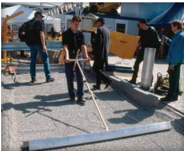
Figure 25. Manually screeding the No. 8 stone setting bed.
