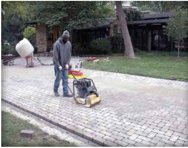
Figure 19. Plastic edge restraint is spiked into the dense-graded base berms so it can hold the pavers in place during compaction and service.
