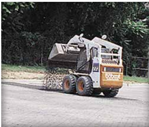
Figure 29. Various methods of filling and sweeping PICP joints.
