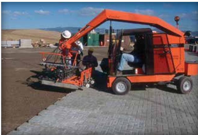
Figure 1. Mechanical installation of interlocking concrete pavements (left) and permeable units (right) is seeing increased use in industrial, port, and commercial paving projects to increase efficiency and safety.
