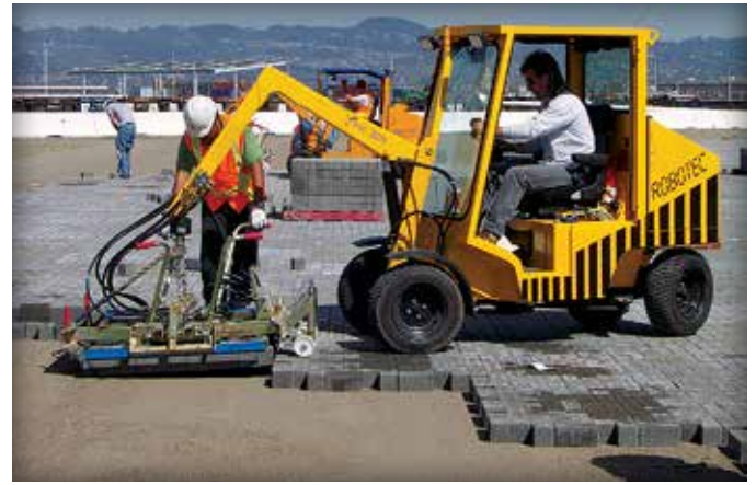
Figure 4. Hydraulic clamp picking up layer of pavers
