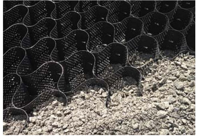
Figure 9. Geocells partly filled with aggregate
