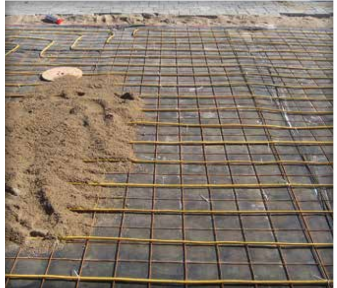
Figure 7. Spreading and screeding bedding sand must be done without moving or damaging pipes or wires for melting snow.
