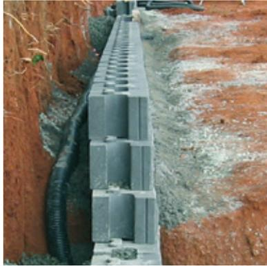
The perforated pipe should be placed approximately 6 inches behind the back of the block. The actual location of the drainpipe should be noted on the engineered shop drawings.
